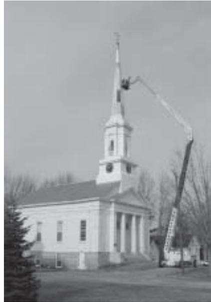
As a matter of fact, both the rebuilding and the fundraising are progressing nicely. Skyline Engineering has slowly stripped and replaced rotted sheathing and support members, working their way around the steeple, from bottom to top, using massive bucket lifts. The entire steeple surface was “wrapped” in a semi-permeable membrane – Tyvek – which allows air to circulate but sheds water. The arrival of large steel sheets was imminent which will
